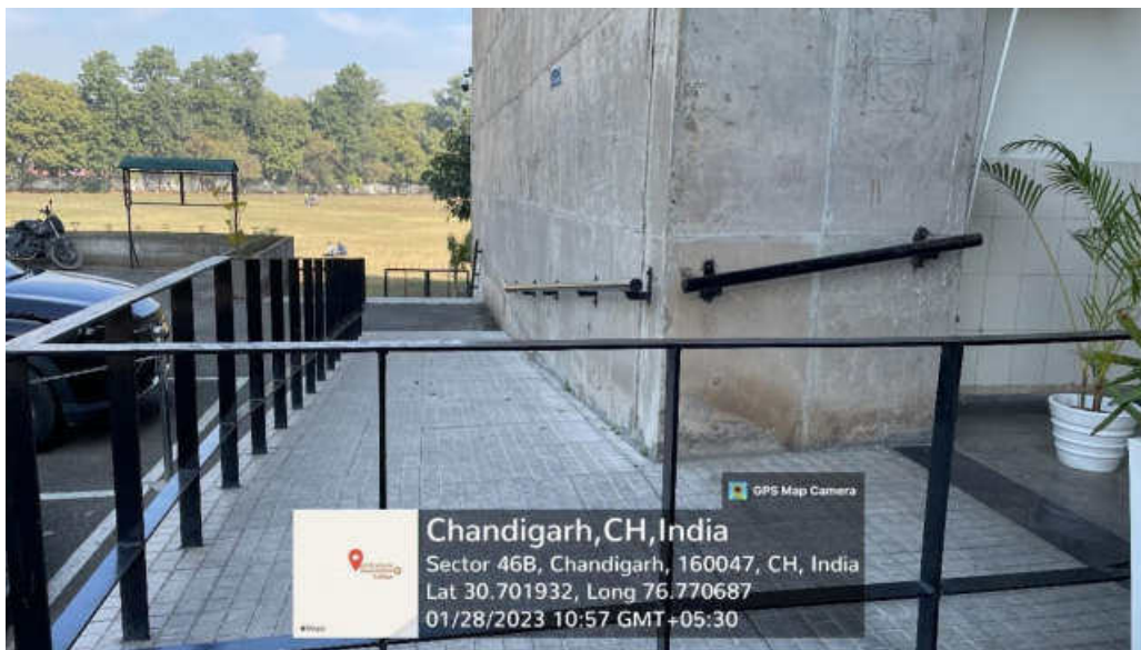
Ramp for Easy Access for the Differently Abled
